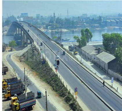
Fig 02:Kanchpur Bridge(Exposure B)
