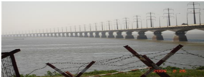
Fig 03:Jamuna Bridge(Exposure C)
