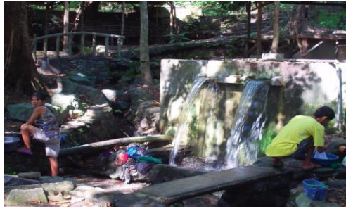
Figure 3. The main concrete water reservoir of Arayat National Park.
