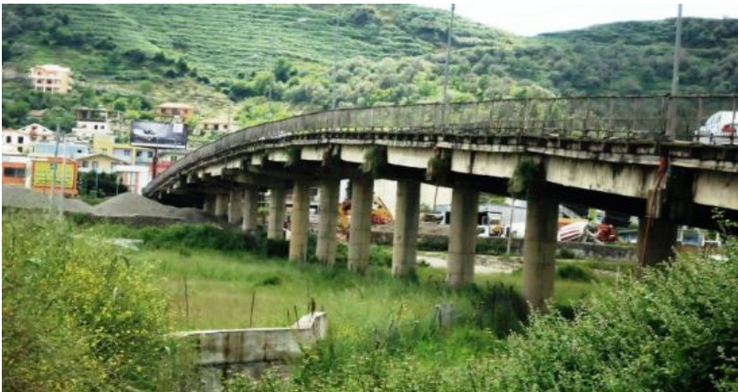
(RC) Bridge columns. Multi – span simply supported concrete girder bridge 1 .
