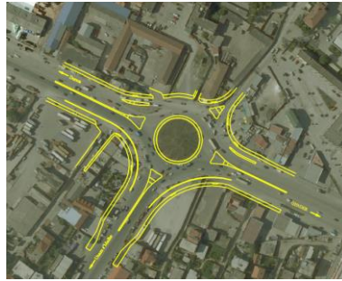
Fig. 1. Aerial photo of the roundabout “Shqiponja”
