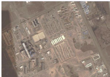
Figure: Shows Kosti power plant project
