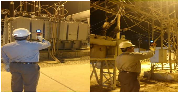
Fig. 4. Infrared Photography by Hot Find LXS model camera from equipments of sample power stations
