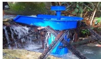
The Installed Pico hydro Electric Generator System
