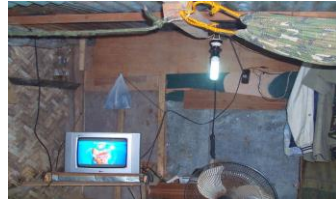
The installed electrical system inside the 703 rd brigade military barracks
