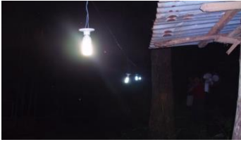
The installed park lighting system
