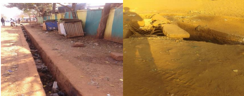
Waste materials in side drains
