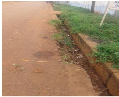
Severely failed side drains
