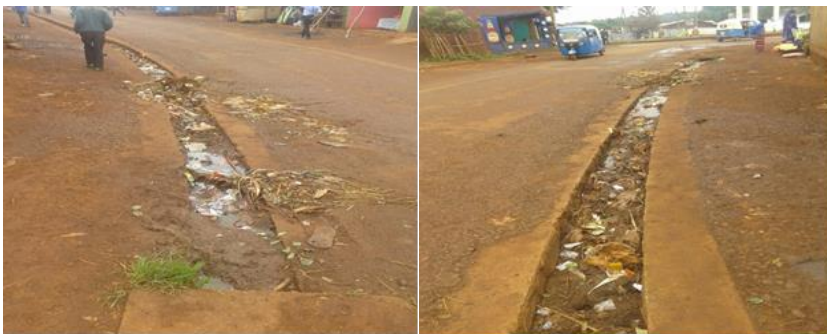
Fully Blocked Drains
