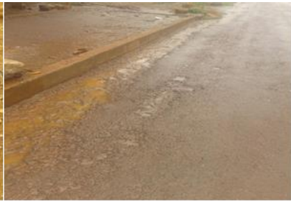
Eroded pavement surface
