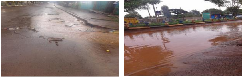
Figure 1: Ponding of water during rain on road surface near to Assosa town Administration Office
