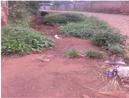
Drains covered by Grass
