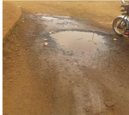
Potholes on Road Pavement
