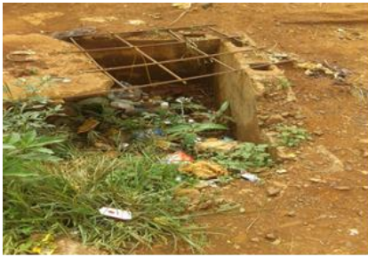
Failed manhole
