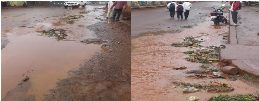
Street Flooding because of drains blockage
