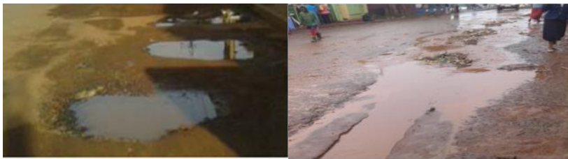
Figure 5: a) Ponding of water on potholes b) Surface Runoff on road pavement
