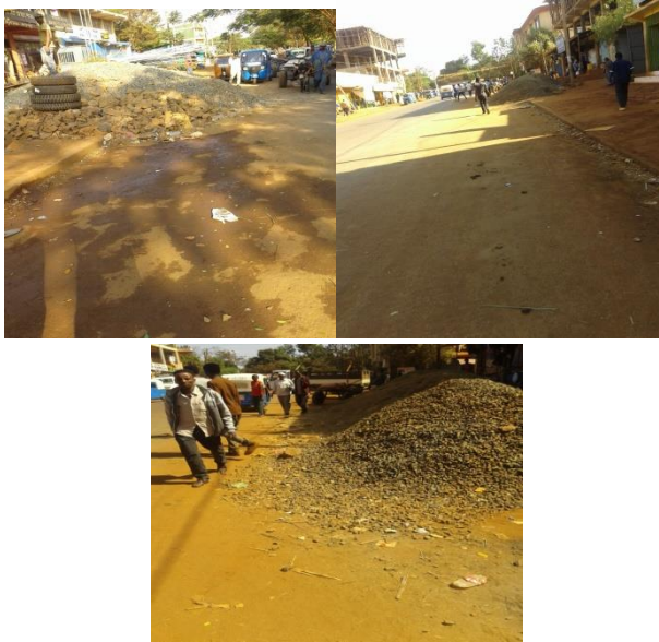
Figure 5: Illegal Encroachments on sidewalks by building materials
