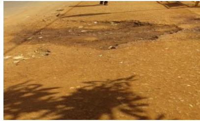
Potholes on Sidewalks
