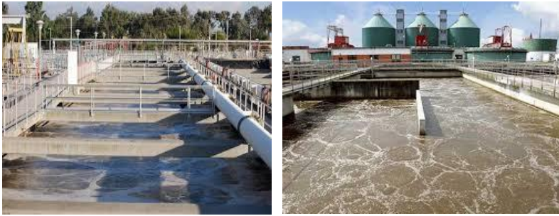
Figure 3. Real Waste water treatment plant
