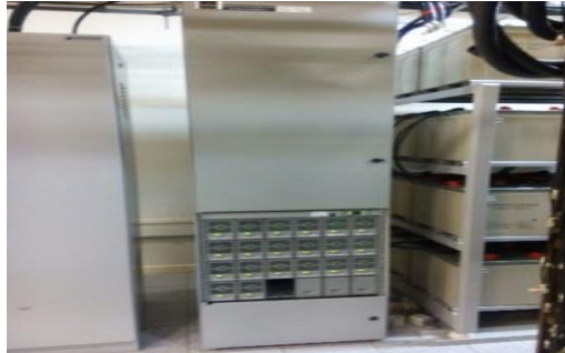
Figure 7-DC Power System Serving a Telecom Station.
