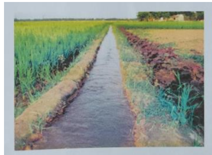
Figure 5: Finished improve earthen canal
