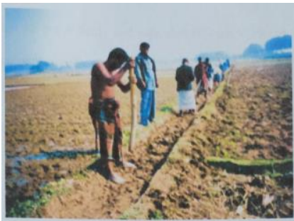
Figure 4: Preparation of improve earthen canal
