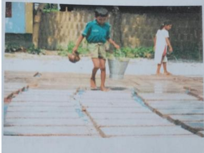
Curing of pre-cast rectangular slab
