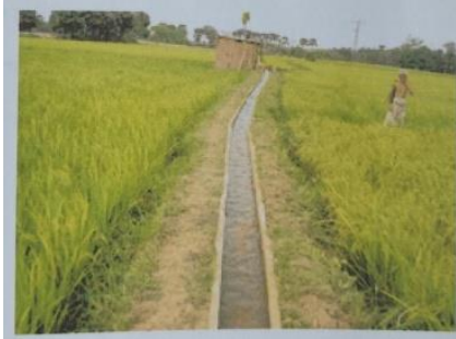
Finished pre-cast rectangular canal
