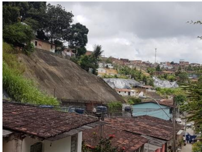
Figure 8: Buildings along the slope.
