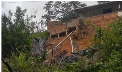
Figure 7: Discharge of sewage directly into the ground.
