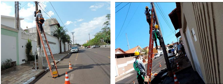
Figure 1 – Installation of Fiber Optics
