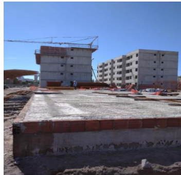
Figure 2. Construction of raft
