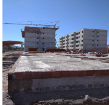
Figure 2. Construction of raft
