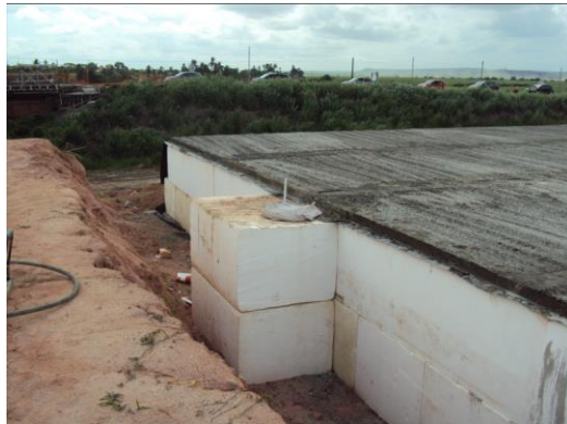
Figure 3 – Use of EPS at BR 101 highway, GOIANA-PE
